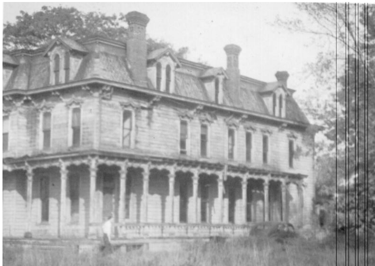
Raymond Stone surveys his recent purchase – circa 1947. This photo shows the complete house prior to the back section being removed.
